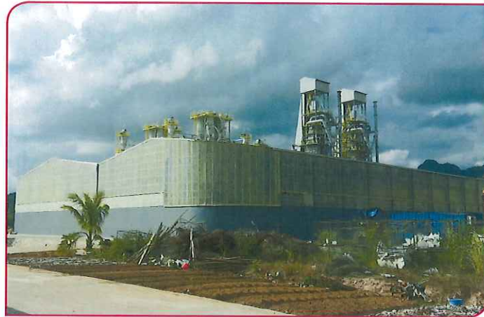
Right and below: The Huong Hai Group lime plant in Vietnam has undergone commissioning.
